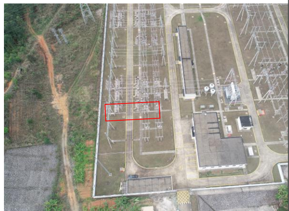
傍浦变电站扩建间隔
