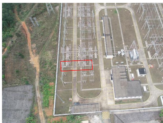
傍浦变电站扩建间隔
